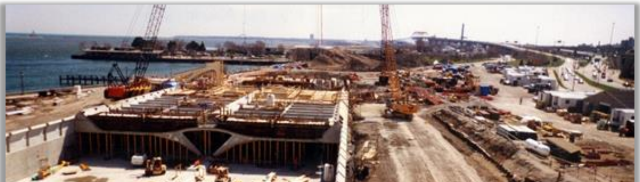
Construction of the Milwaukee Art Museum | Quadracci Pavilion, circa 1999
